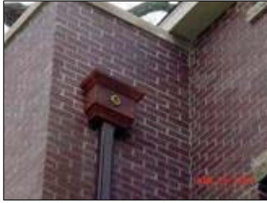
Copper collection box and downspout.
