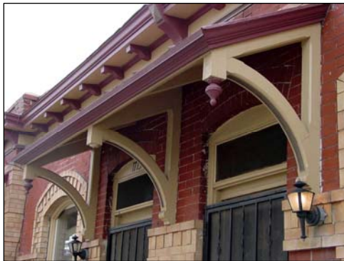
Example of decorative roof-wall junction.
