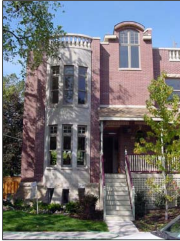
Mixed materials including brick/limestone walls with painted cedar porch on row house building.
